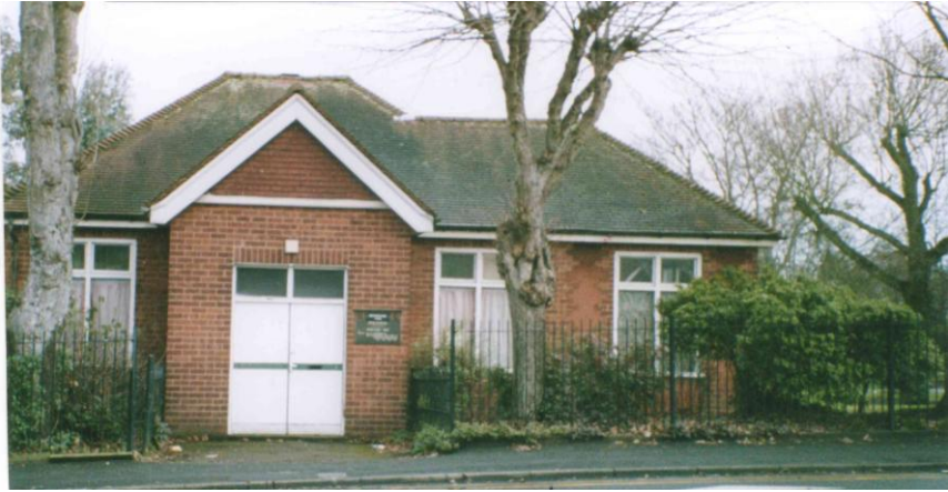
Sons of Rest Pavilion as it is today in Sutton Road
