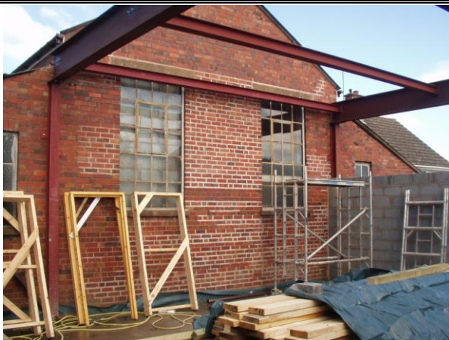
Extension in progress (early 2005)
