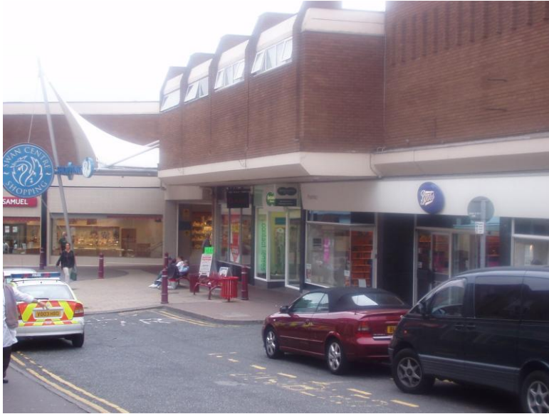
The same scene today – the site is occupied by the Swan Centre and by Specsavers
